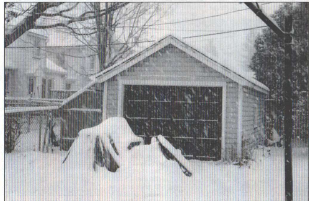
CARDIO in COLD STORAGE ... (under the tarp) outside the 1926 wood frame detached 20' x 12' garage.
